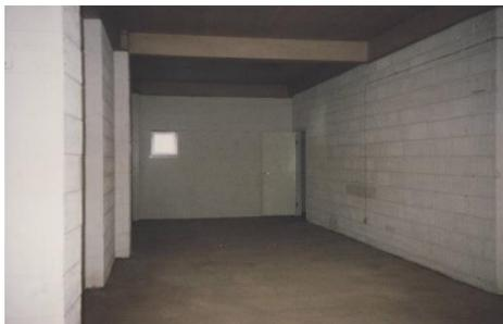
Laying a smooth, concrete floor was the first stage.
